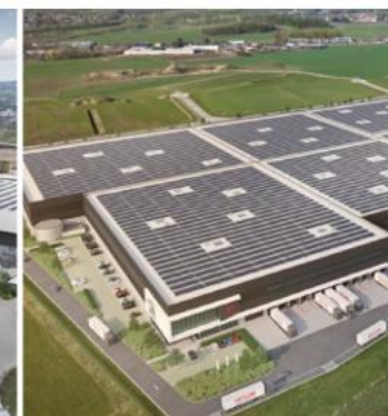
Logistics Campus 21 - Q1 2026 - Heylen Warehouses - 110,000 m 2
