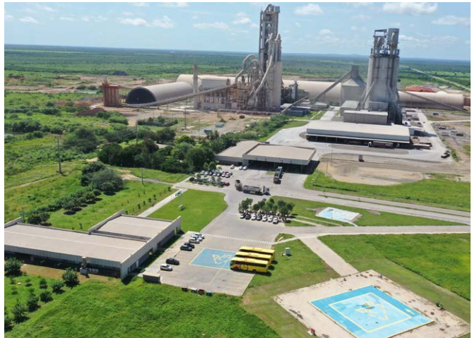
Quixere cement plant, Brazil
