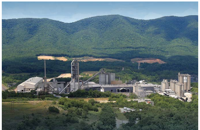
Roanoke cement plant, USA
