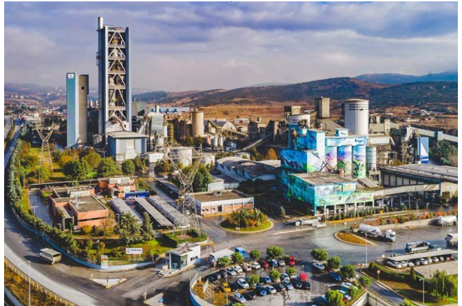
Thessaloniki cement plant, Greece
