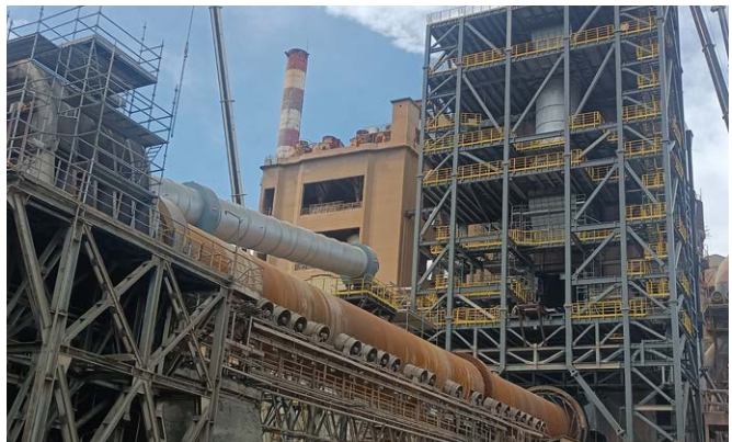
Pre-calciner unit under construction in Kamari plant, Greece
