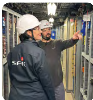
Christelle, project manager, and Paul, electrician.
