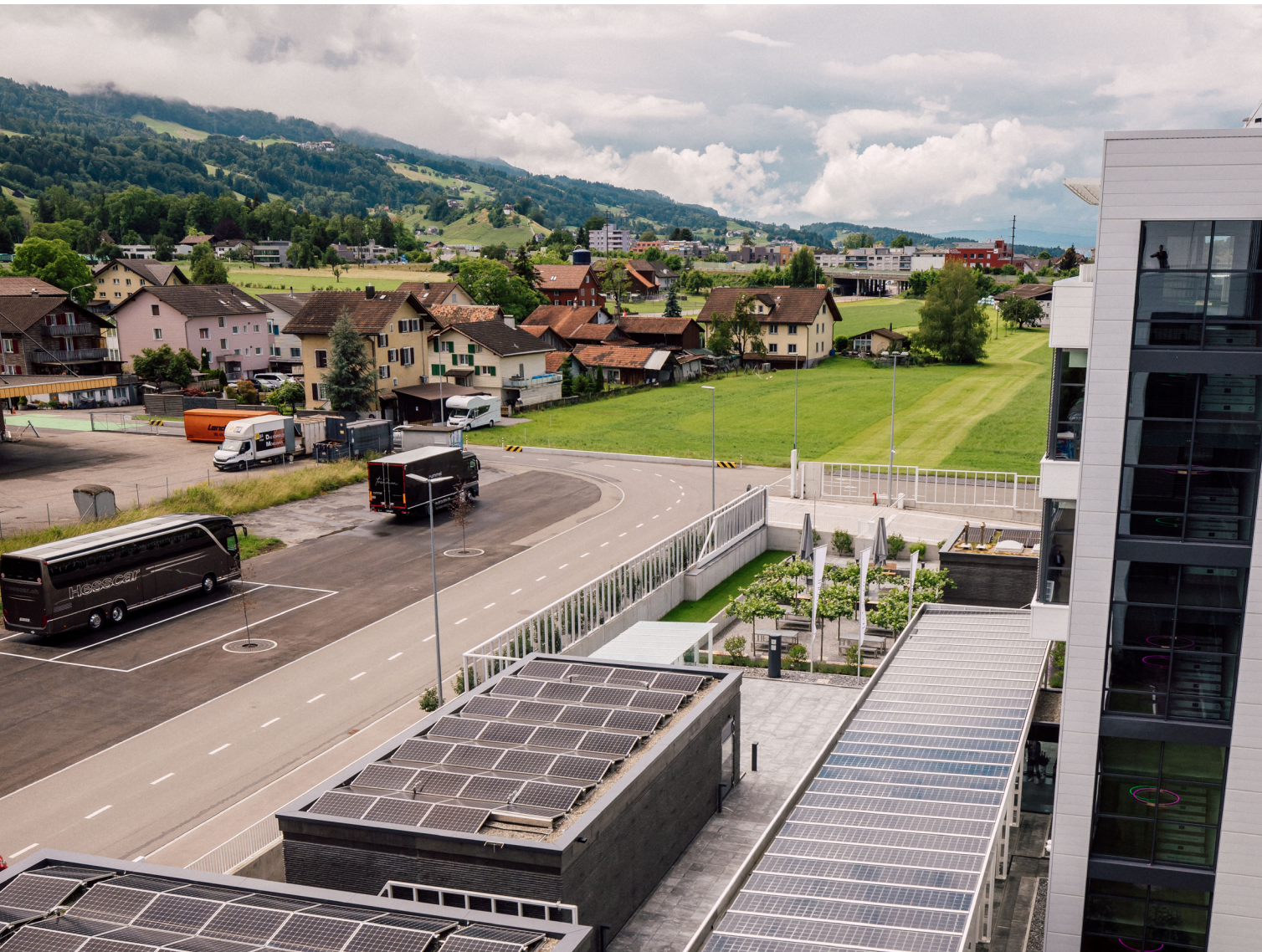
ELC's Galgenen Distribution Center in Switzerland.
