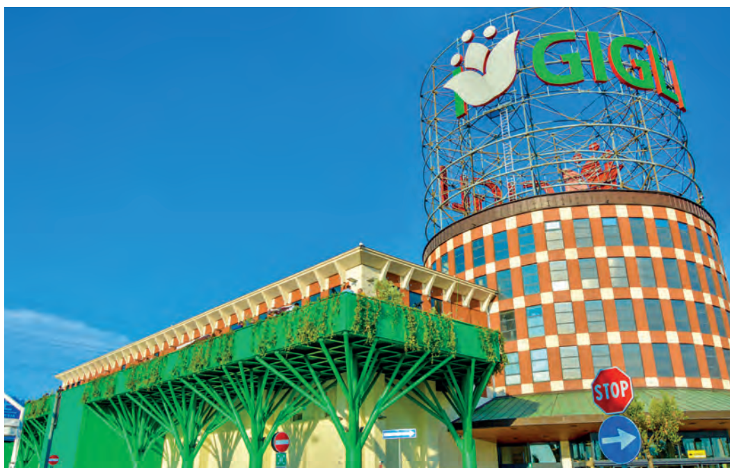
The new terrace at I Gigli.
