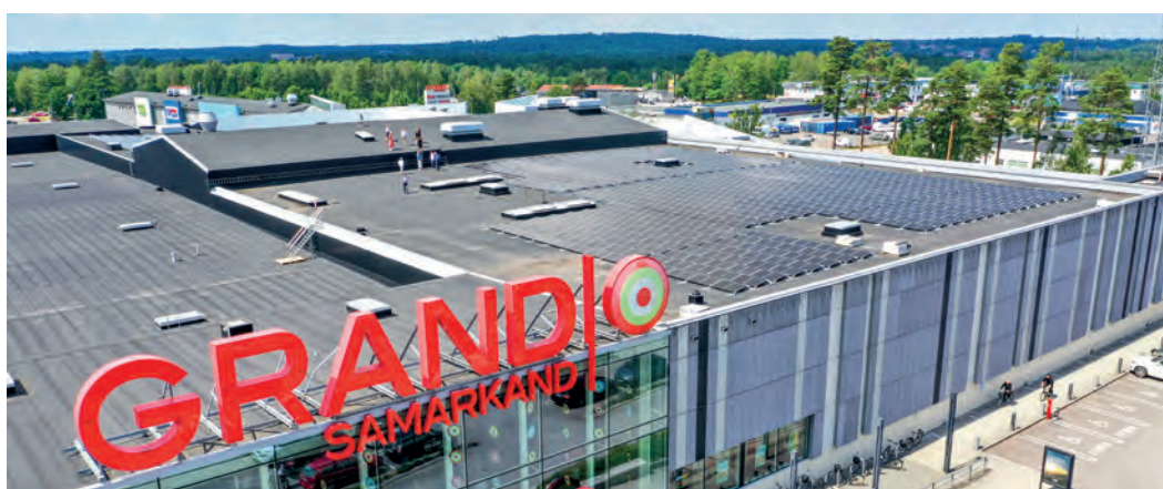
Solar panel roof installation at Grand Samarkand.
