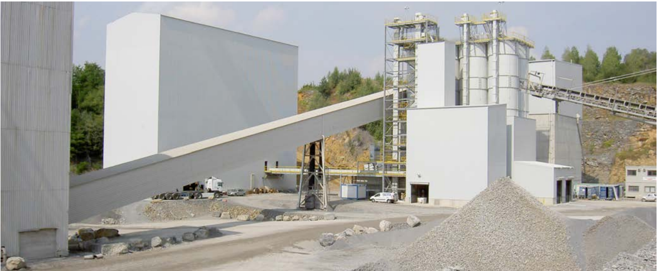
Housing around installations, using insulating boards
