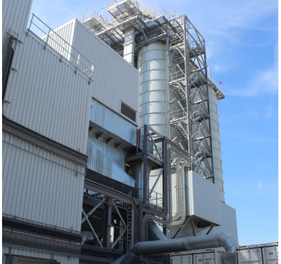
Our new filter installation in Aisemont, Belgium
