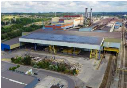
Châtelet (Belgium) Melt shop and hot-rolling mill
