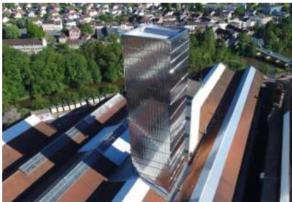
Gueugnon (France) Cold-rolling mill and finishing facilities
