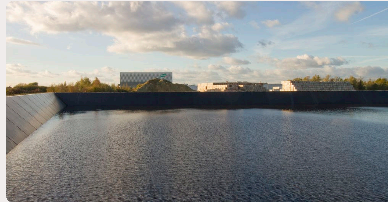
In Ardooie, the purified waste water from the Ardo site is pumped into a 150 million liter reservoir
