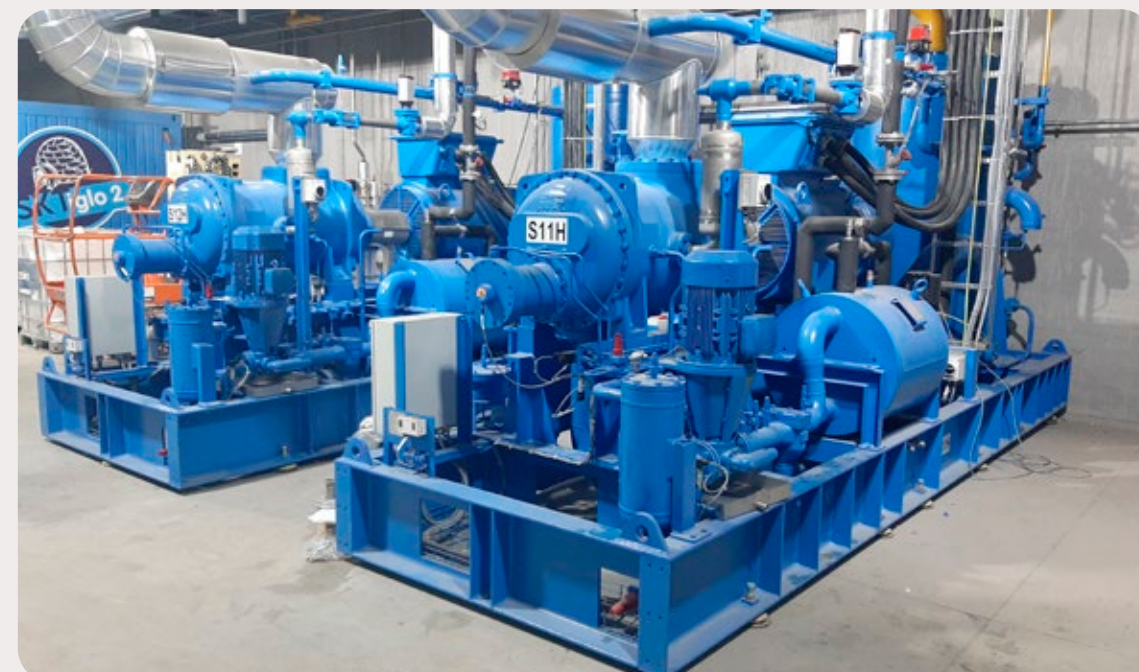
Capturing the residual heat from the cooling oil in our compressors to generate warm water for cleaning purposes
