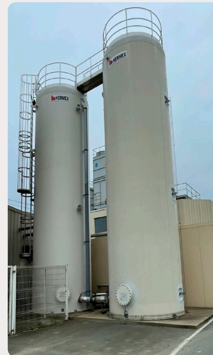
Two water tanks of 75m³ at our site in Gourin, to store the site's hot water. The water is heated with residual heat
