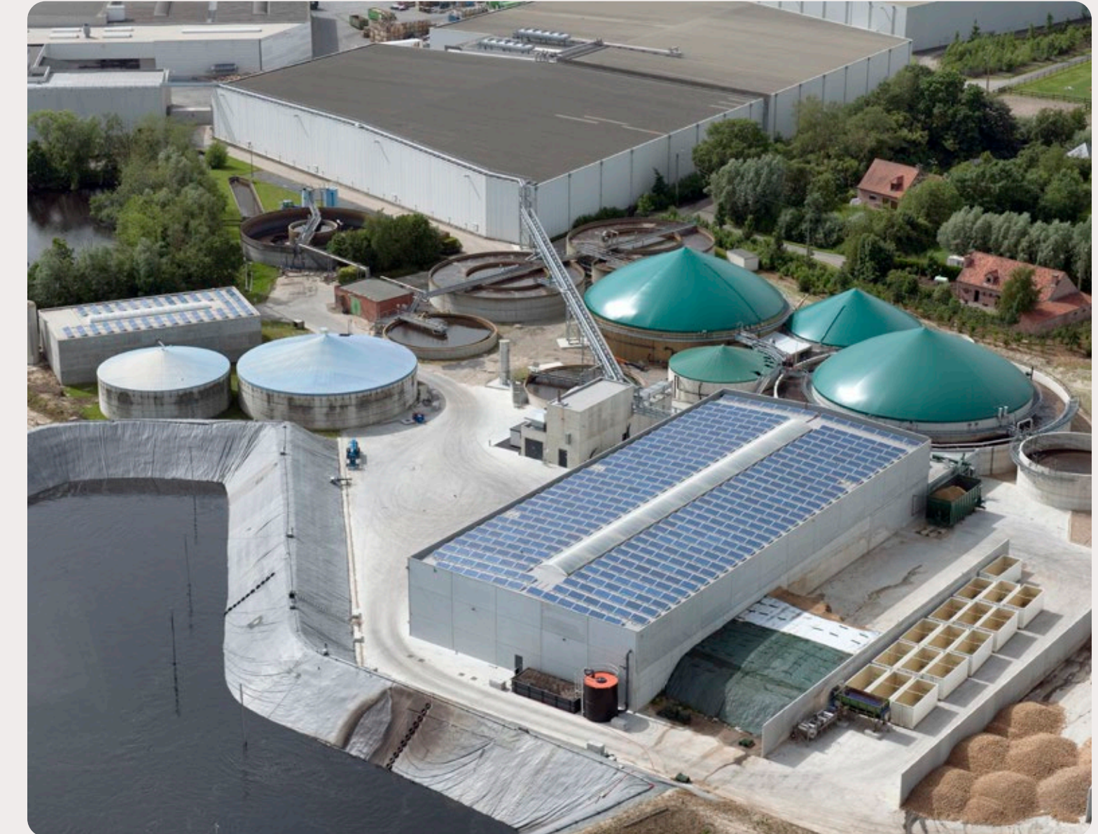
Green electricity and green steam generated at the biomethanisation plant in Ardoeie (BE)
