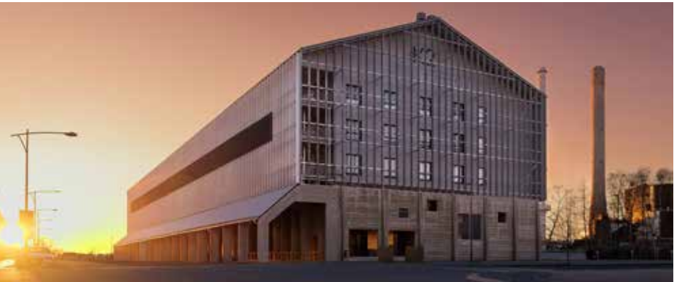
OULU SATAMATIE 34 - SERVICE COMMUNITY IN OULU (FI)
