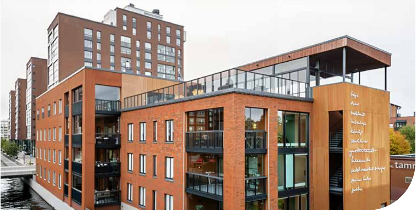
TAMPERE KANAVANPORTTI - CARE HOME IN TAMPERE (FI)
