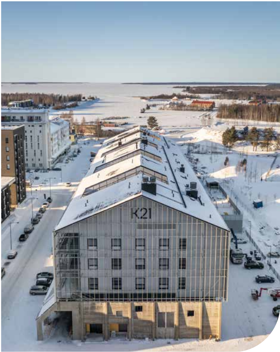
OULU SATAMATIE 34 - SERVICE COMMUNITY IN OULU (FI)
